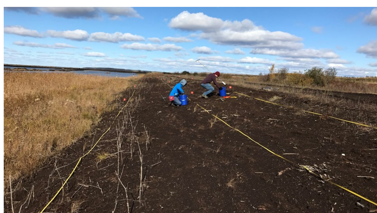
Figure 1. Harvested slope area.
