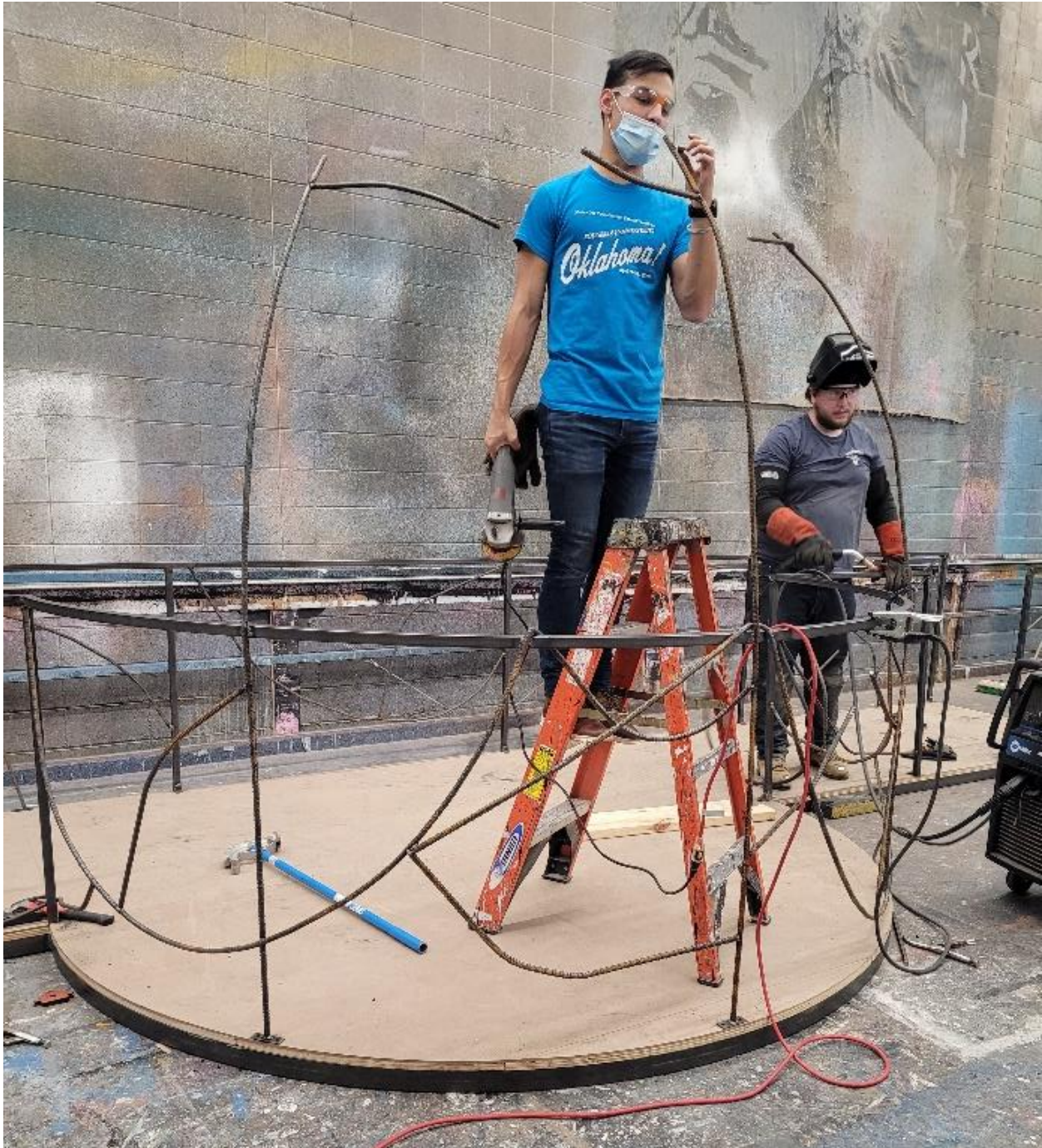
A work-study student inspects to ensure there are no sharp edges
