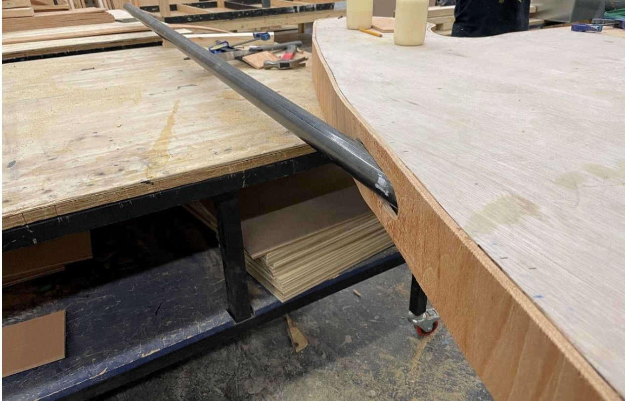
An opening cut into the bending plywood to allow for the steel beam
