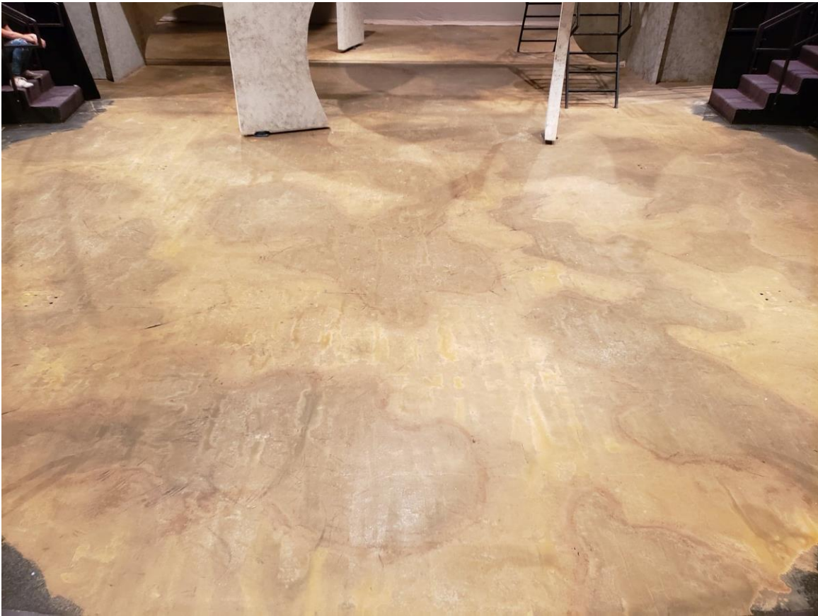
Figure 81: Final paint treatment
