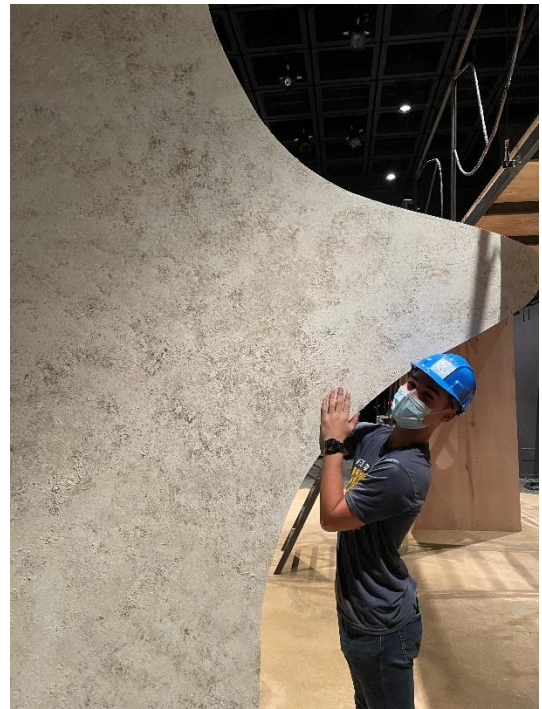
Figure 76: Finished wall treatment
