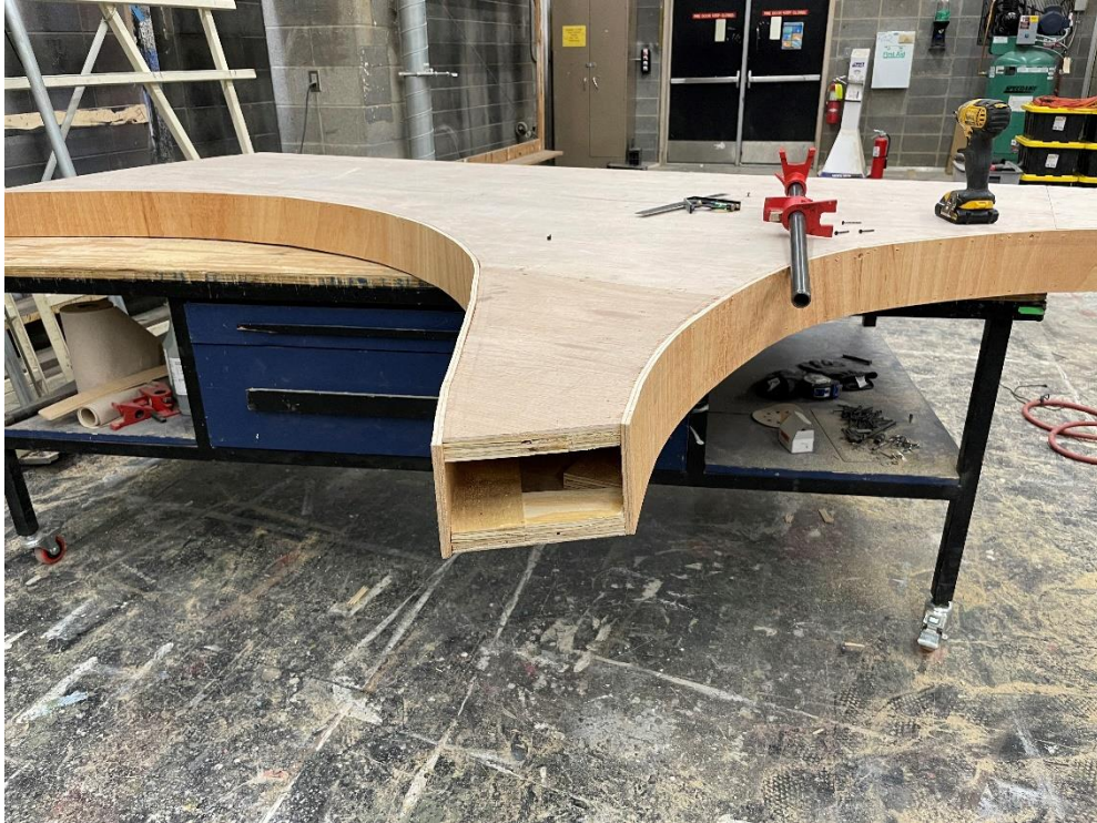
Figure 71: Attaching the bending plywood
