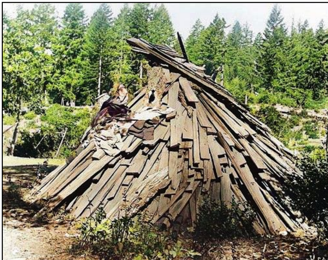
Nongatl conical house near Blocksburg, 1903. The traditional bark cladding has been replaced by small pieces of milled wood (CEFP, colored by JR).
