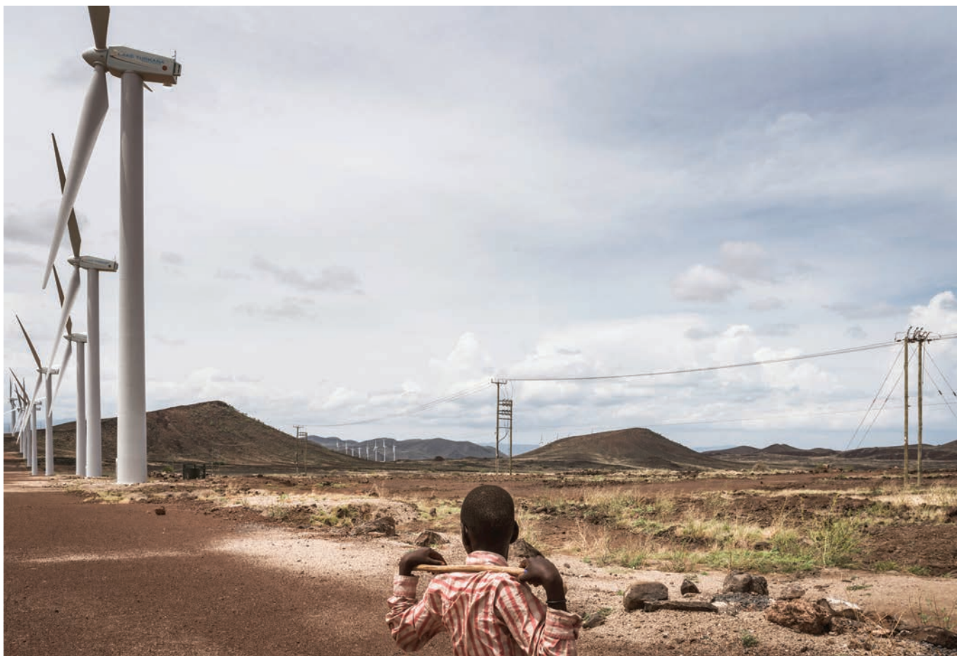
Lake Turkana wind power installations, Kenya.
