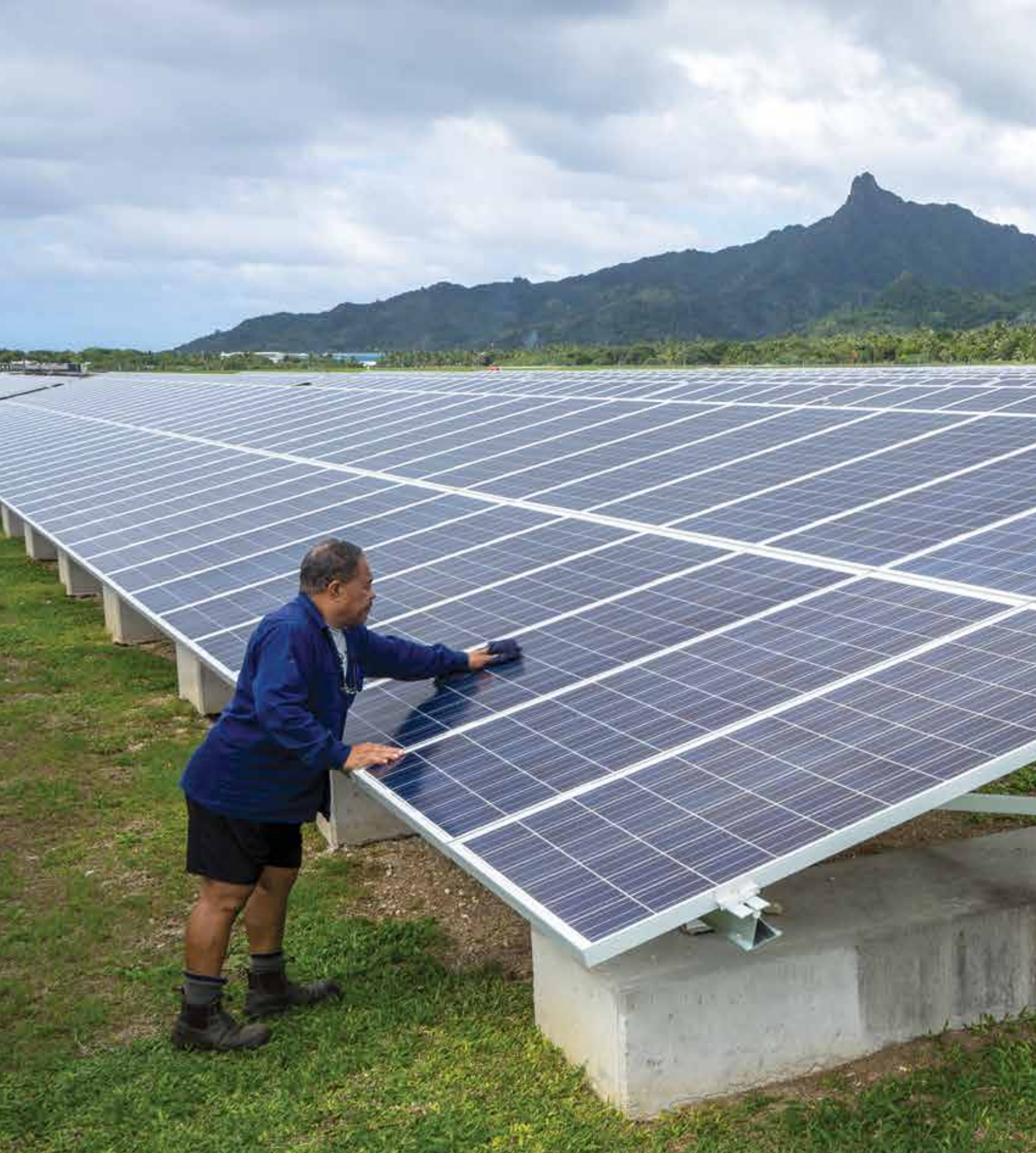
Solar power in the Cook Islands. ADB's Renewable Energy Project aims to reduce the Cook Islands' heavy reliance upon diesel fuel for electricity generation by funding solar power plants on six islands. The transition to solar energy should reduce diesel-fuel consumption by 1 million liters per year (photo by Eric Sales/ADB).
