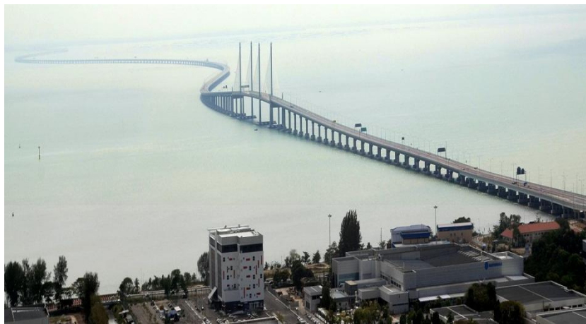
Figure 1. Overall view of Penang second bridge.
