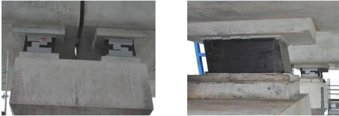
Figure 2. Location of the rubber bearings in Penang second bridge.
