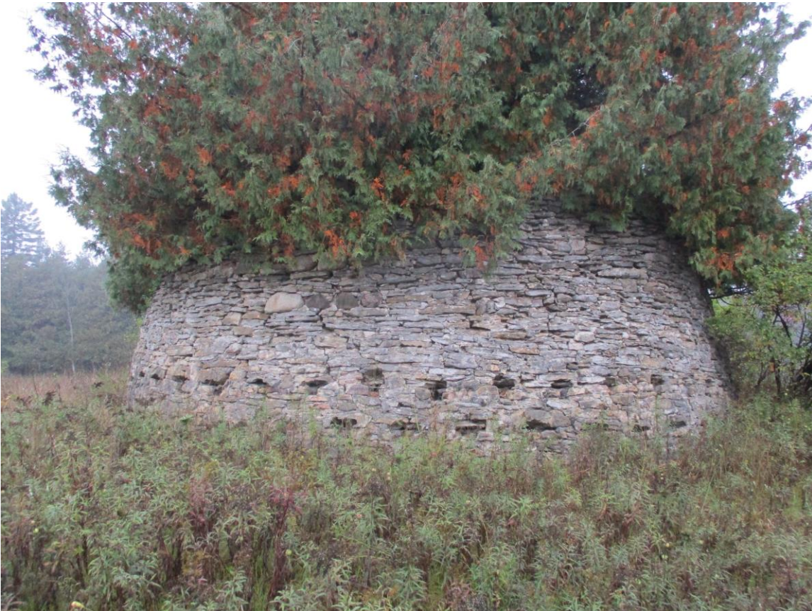
Tree growing from top of a Wilson charcoal kiln, 2021. Unfortunately, trees are growing out of many of the remaining kilns around the Upper Peninsula.
