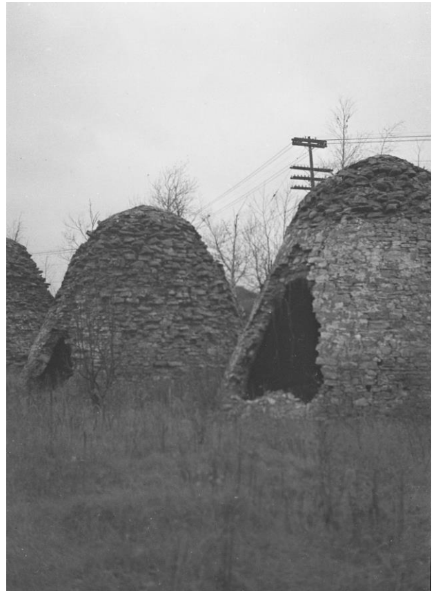
The Carp River kilns as they sat along the highway. Credit: Superior View.
