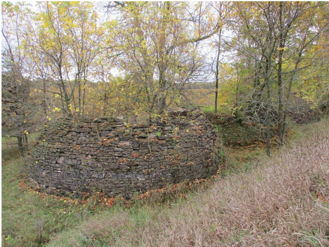
Stephenson charcoal kilns in a row near an embankment for top loading, 2021.
