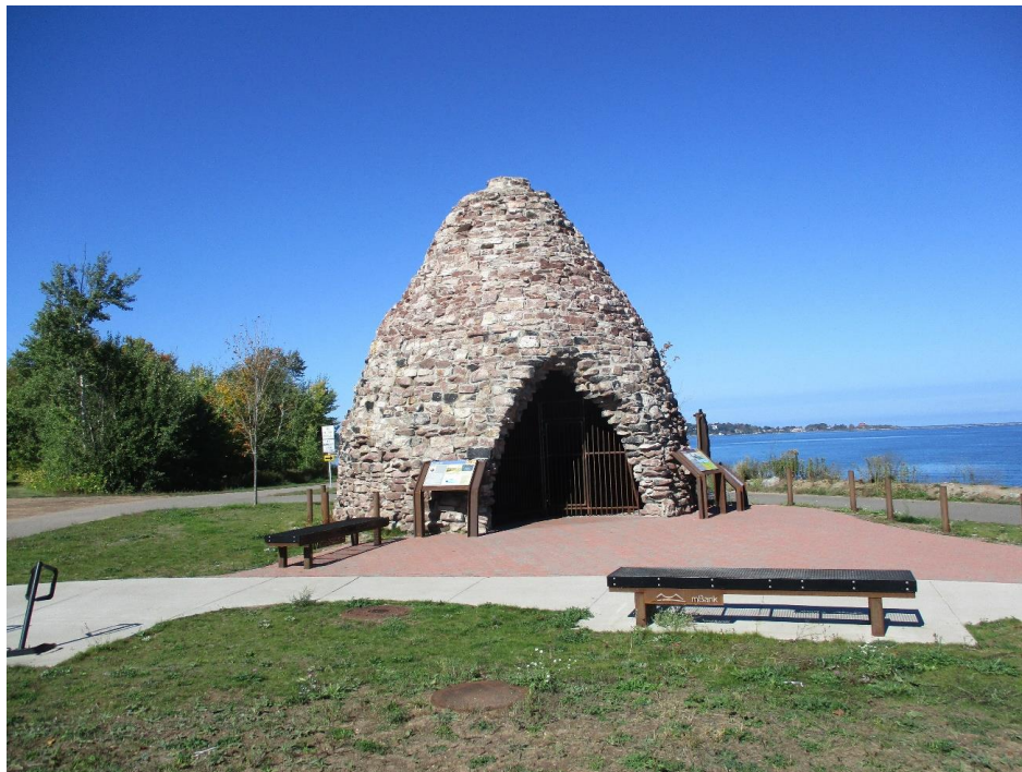
The restored charcoal kiln in 2021 stands on the north side of the Carp River on U.S. Highway 41, very close to the site of the old kilns, and welcomes visitors to Marquette by celebrating the city's mining history.
