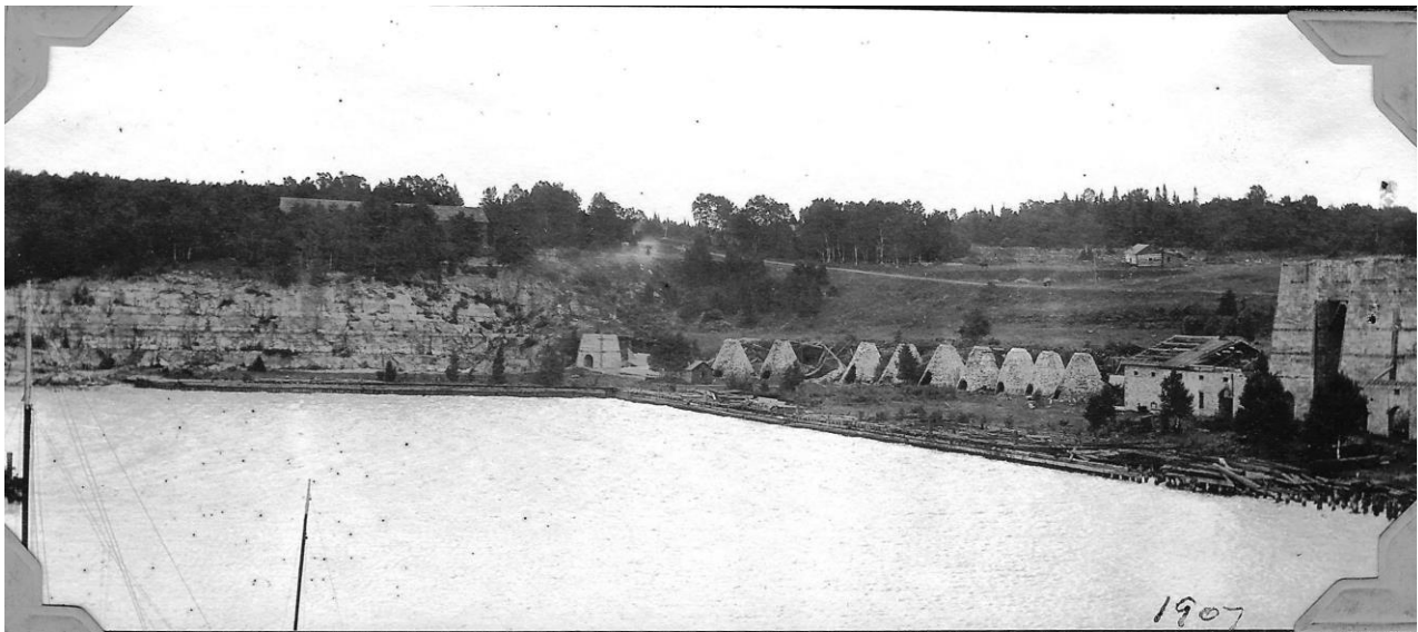
The charcoal kilns in a row next to the furnace at Fayette about 1907. Credit: Delta County Historical Society.
