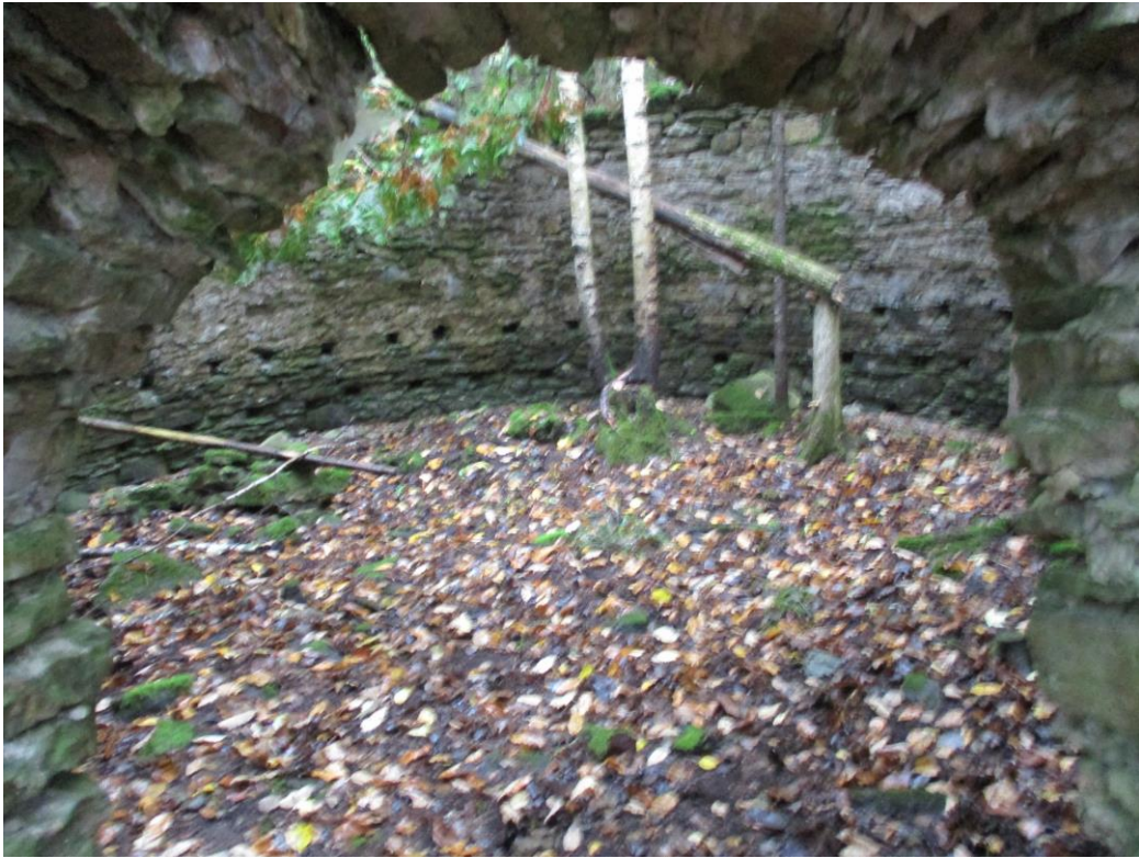
The bottom door and inside of a Bark River charcoal kiln, 2021. Notice the rows of air vents.
