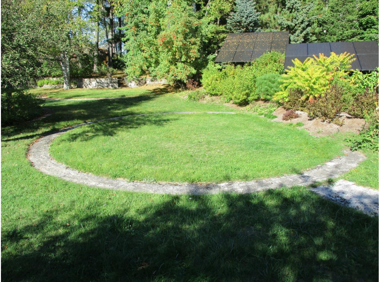
Charcoal kiln foundation on Lakewood Lane in 2021 as it stands in the yard.
