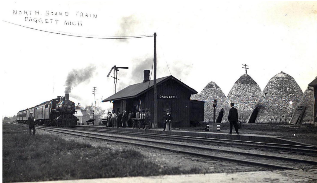
Charcoal kilns were often at railroad sidings or very close to railroads to minimize transportation cost in getting the charcoal from the kiln to railcar. These kilns were at Daggett in Menominee County, late nineteenth century. Credit: Menominee County Historical Society
