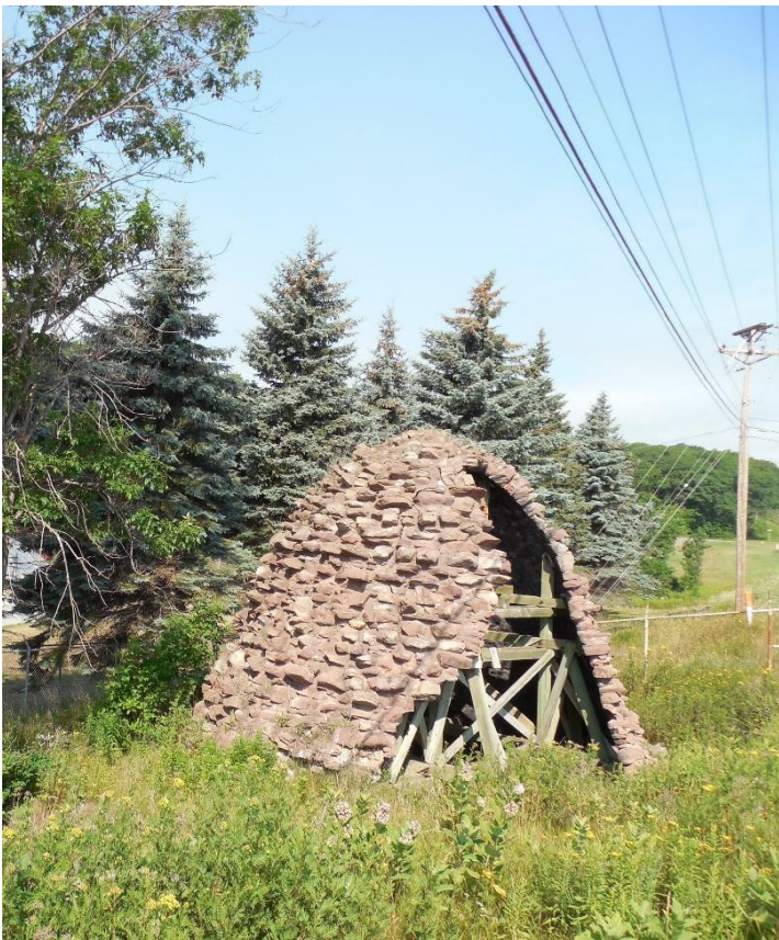
The last surviving Carp River Furnace charcoal kiln along U.S. Highway 41 in 2014. Credit: Jimmy Emerson, DVM, Creative Commons license CC BY-NC-ND 2.0.
