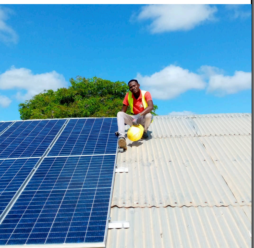
Figure 7. Installation of solar panels on the hospital in Lawra.
