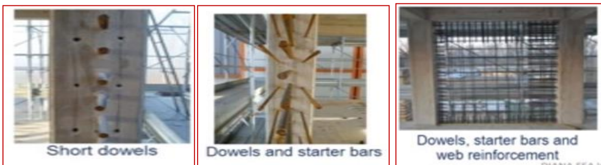
Figure 10. (a) Short dowels- (b) starter and dowel bars, (c) Starter, dowel and web bar
