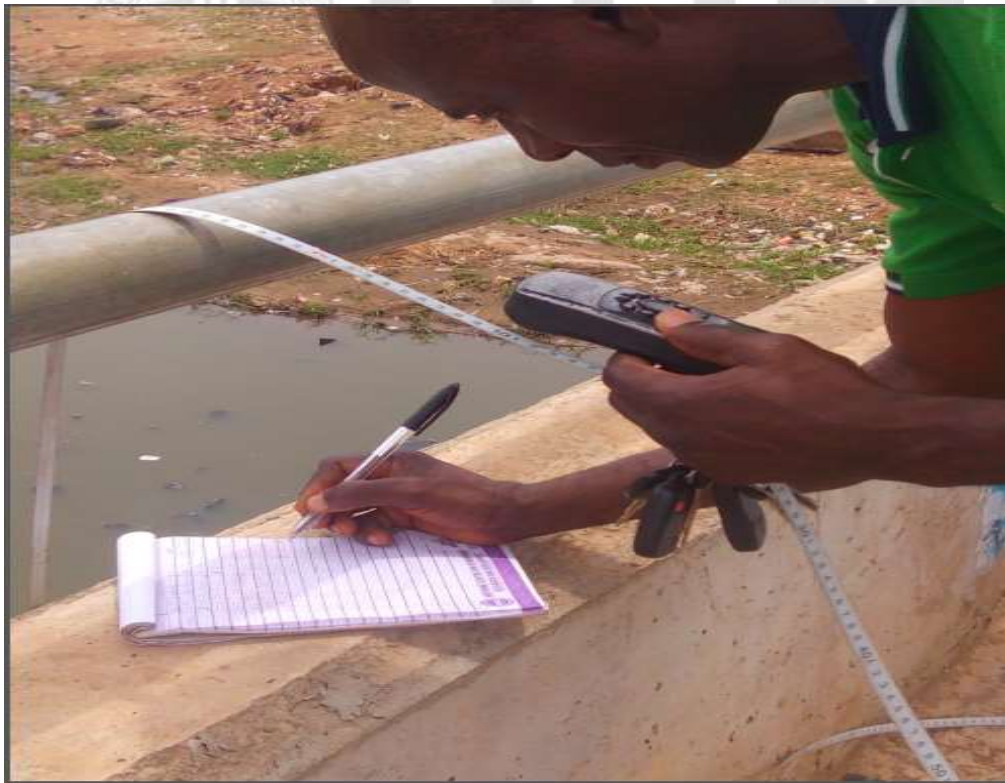
Figure 1.2: Taking the Coordinate Points on Site
