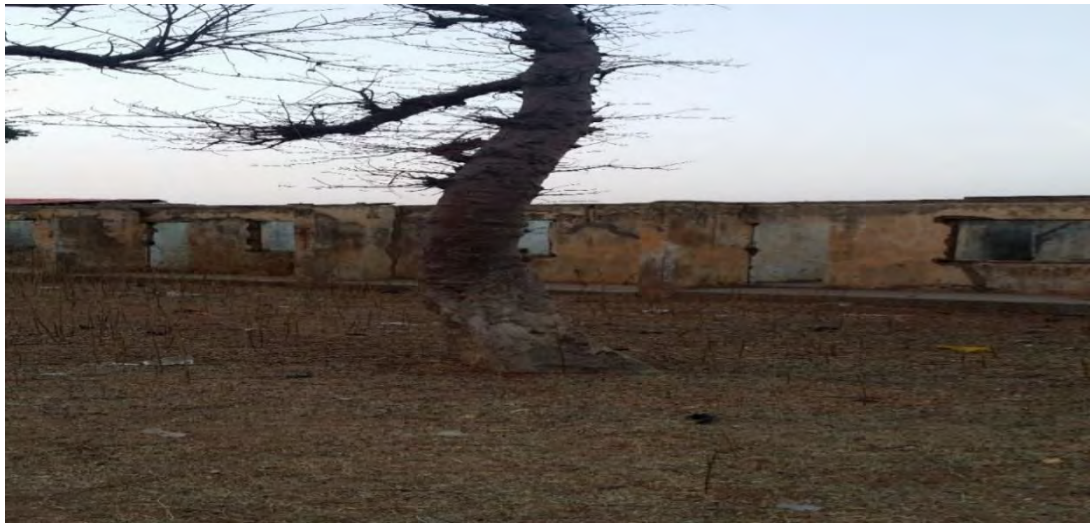
Figure 4.17: Abandoned Primary School in one of the Local Government Areas. Source: Fieldwork, 2018.
