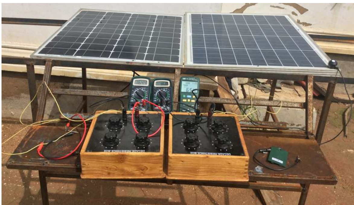
Figure 3: Outdoor PV modules testing
