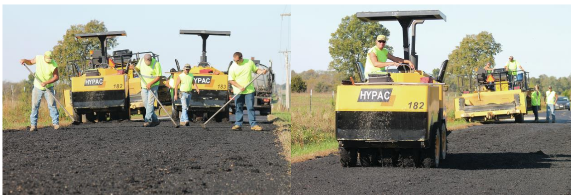
Figure 5. Field implementation of rubberized chip seal with 100% crumb rubber replacement ratio.
