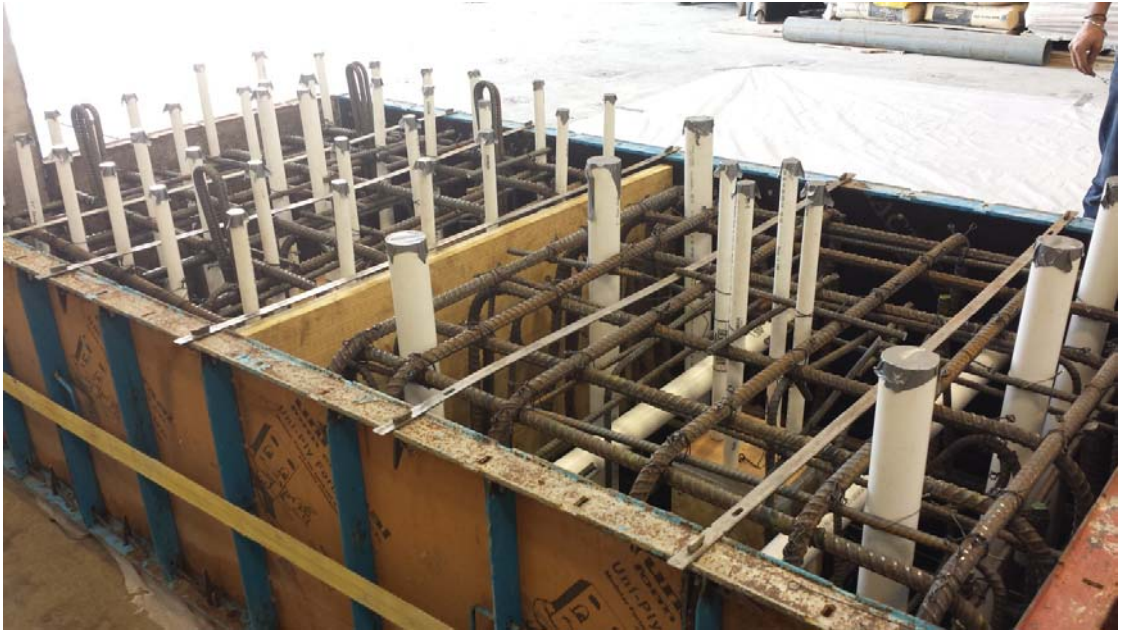
Figure B.4. Foundation and head steel cages ready
