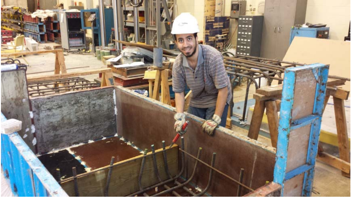
Figure B.3. Foundation steel cage preparation
