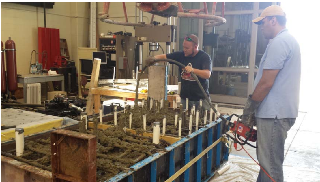
Figure B.5. Foundation and head concrete pouring
