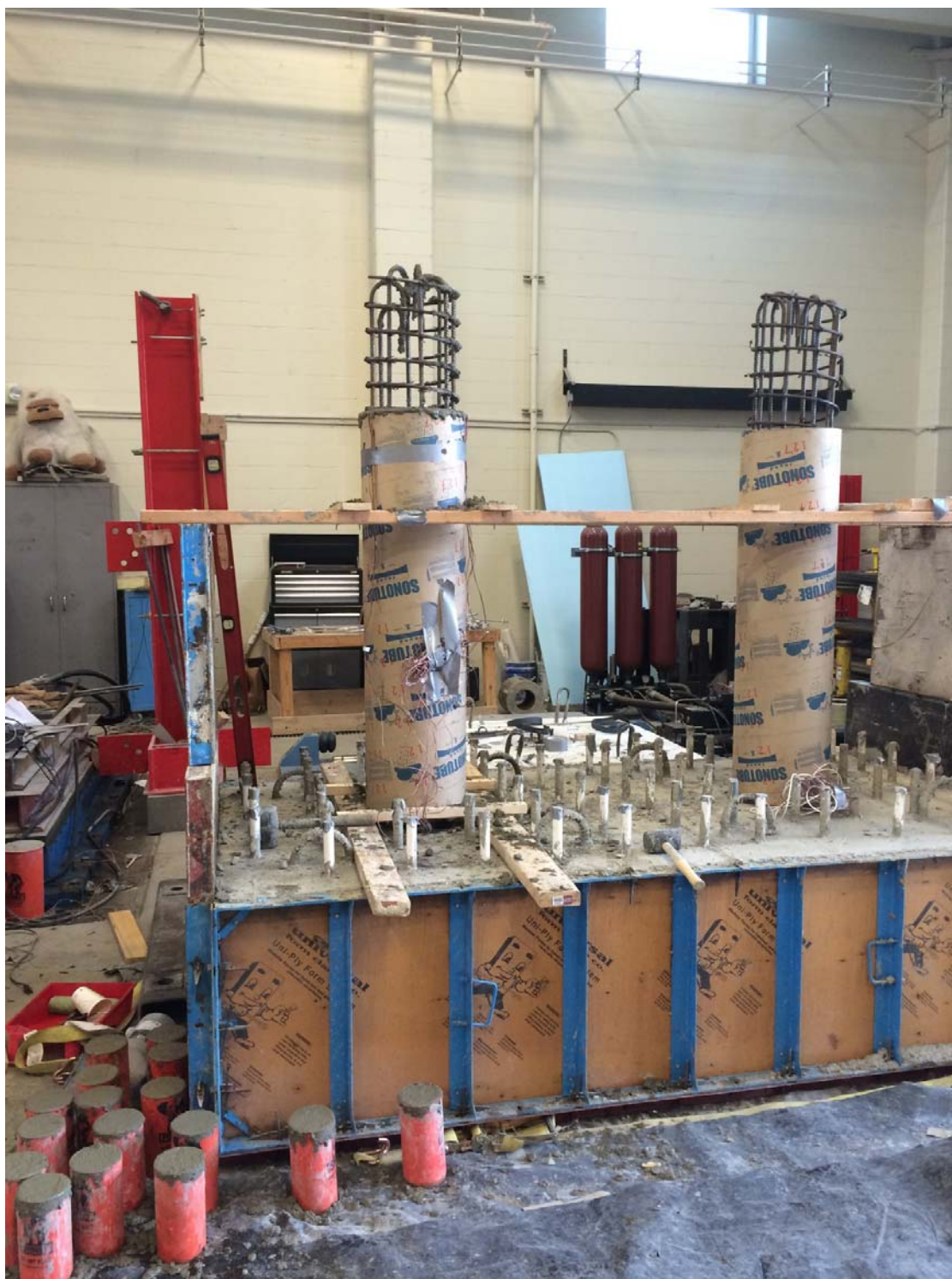
Figure B.9. Concrete pouring for the RC and rubberized columns
