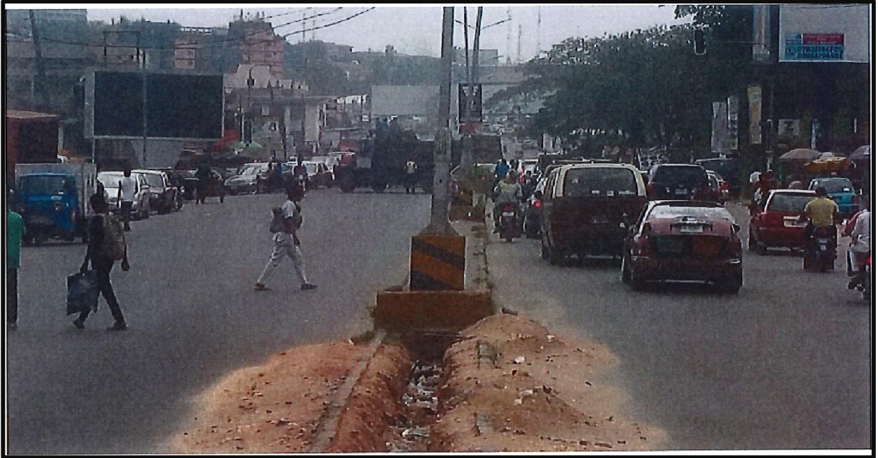
FIG 11 Pedestrians Crossing the road, Dug out Median
