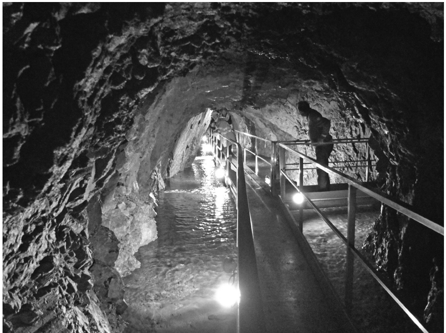
Fig. 8 – Hydrogeological monitoring of Tenda tunnel.
