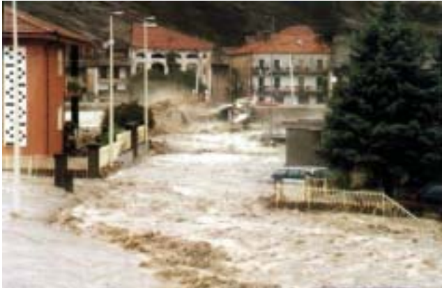
Photo 9 and 10 Hône – Donnas. Dora Baltea river flooding ( author: local media ).
