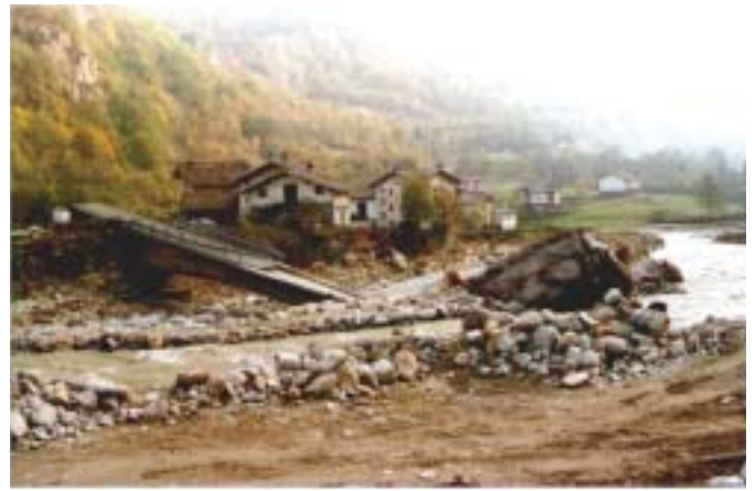
Photo 13 Issime. Lys torrent – Flood effects.
