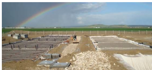
Chorefech (Tunisia) CW WWTP under construction in 2008
