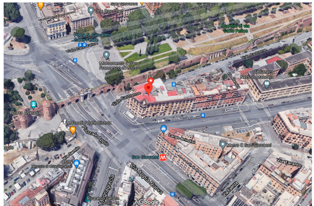
Figure 6. View of the analyzed building on the map, at the intersection of Via Emanuele Filiberto and Via Castrense ( https://www.google.it/maps/place/41%C2%B053'09.2%22N+12%C2%B030'36.6%22E/@41.8835837,12.5093078,320a,35y,39.39t/data=!3m1!1e3!4m5!3m4!1s0x0:0xf6e6a6f12a7bebc20!8m2!3d41.885885!4d12.510169 , accessed on 25 January 2022).
