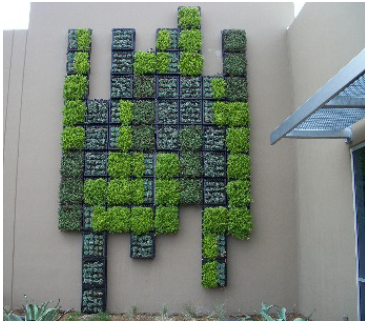
Fig. 3 Panel with soil substrate cells for planting
