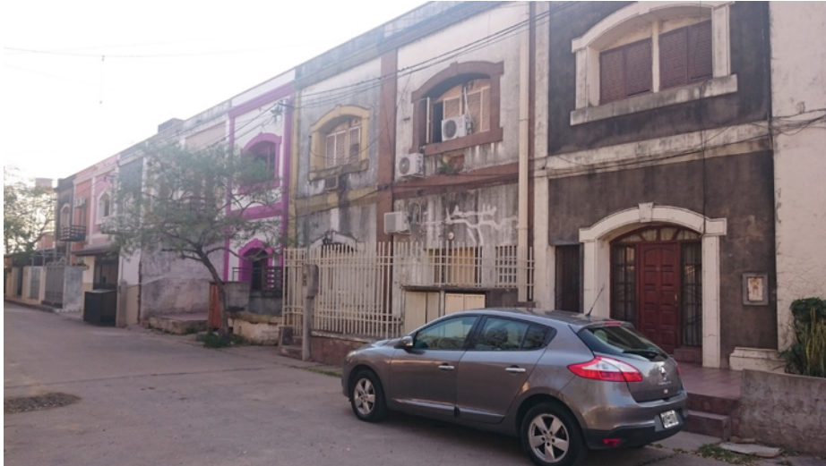
Fig. 8. Housings in the old factory, present state (2018). The sense of individual membership and ownership is clear by the different façade colours, while the new buildings for social housings (see Fig. 10 bottom right) show no sign of individuality.
