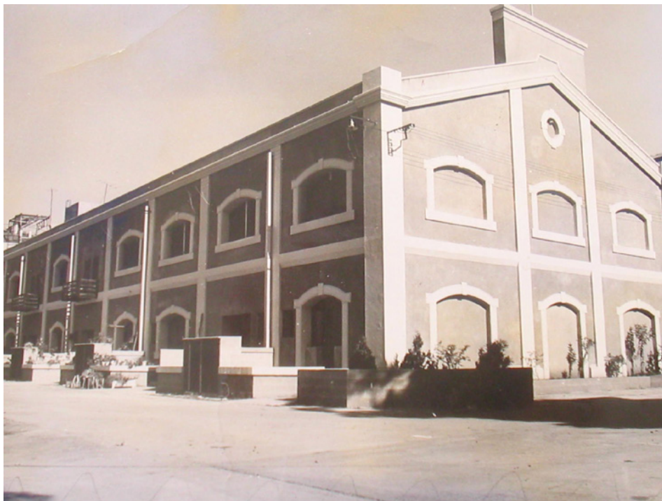
Fig. 6. Apartments integrated into the original factory (photo at the end of the works). All the openings have been respected; only wooden balconies have been added; in front of each entrance a small private garden enhances the sense of privacy.
