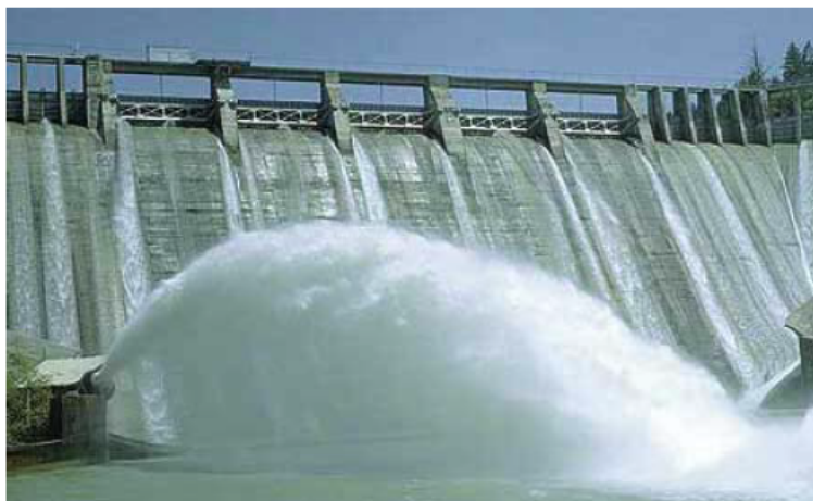
Figure 2.21: Scott Dam, California (Medley 2008).
