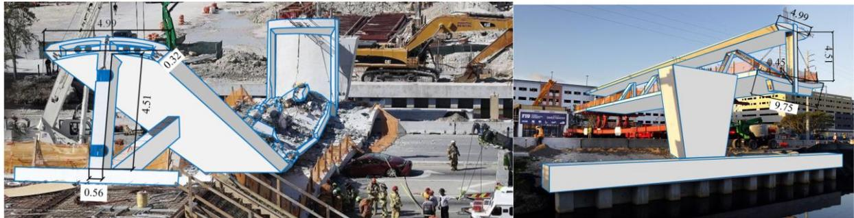
Figure 7 Image-based measurements of the collapsed Florida University pedestrian bridge for forensic analyses (reproduced from Peng et al., 2019).
