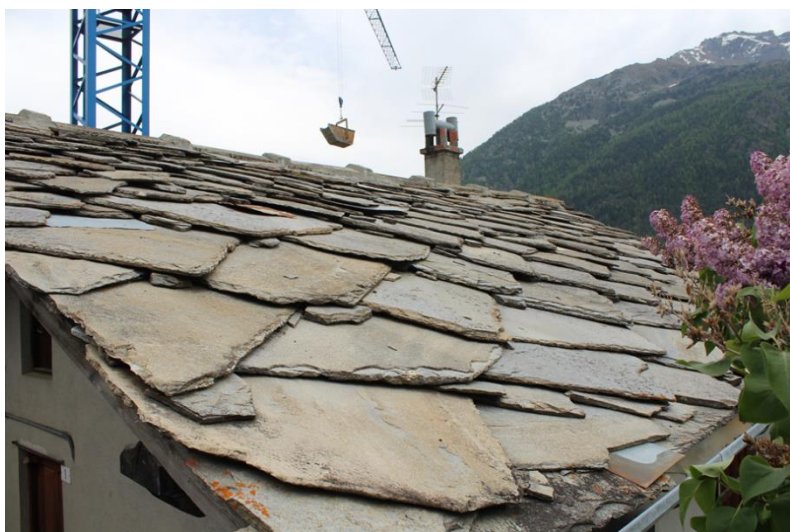
Figure 7. Calcschist CM roofing in Lignod after renovation.
