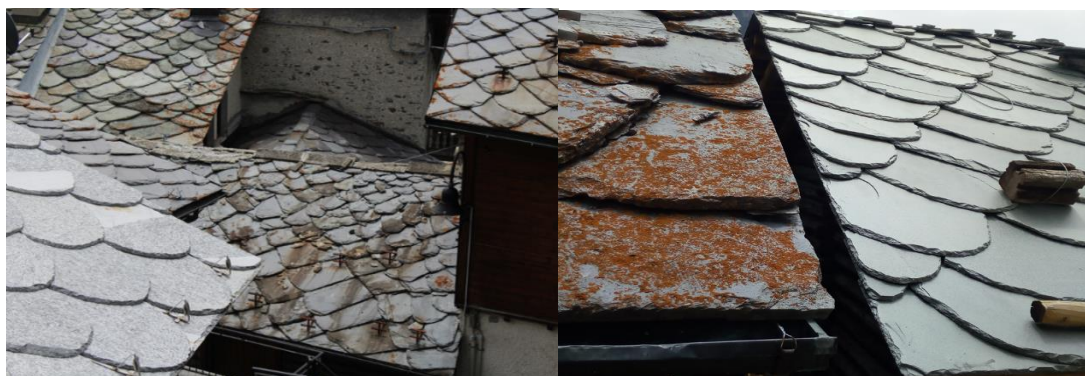
Figure 8. Porfiroide roofing near the new roofs of gneiss on the left and Quartzite on the right in Antagnod.
