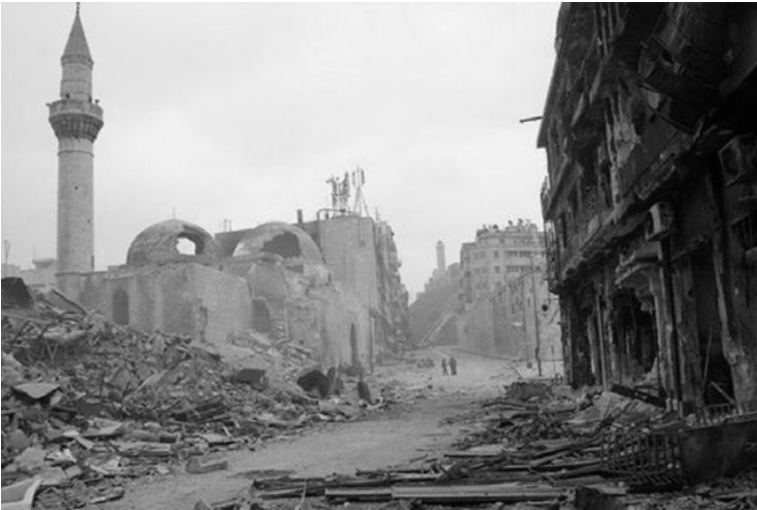
Destructions in Aleppo city, 2014
