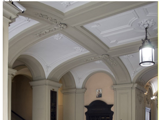
Figure 1. Banded vault in the atrium of the palace in Via dei Mercanti 2 in Turin. Photo: F. Natta
