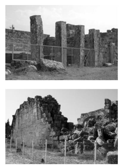
Hierapolis: the Thermae pillars deformed by the earthquake and the walls of the Thermae-Church deformation
