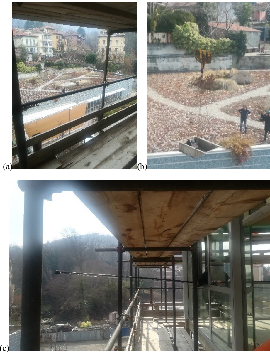
Figure 6.19- (a) first attempt of positioning of the sound source, as seen from inside the indoor environment; (b) repositioning the sound source with the crane; (c) positioning of the outdoor receiver.
