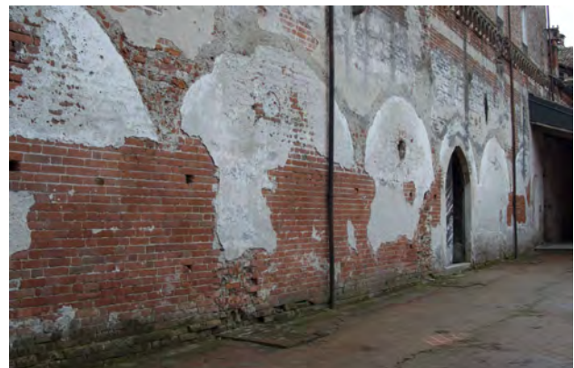
Figure 3. Particular of the refectory entrance (south side of the abbey' cloister)
