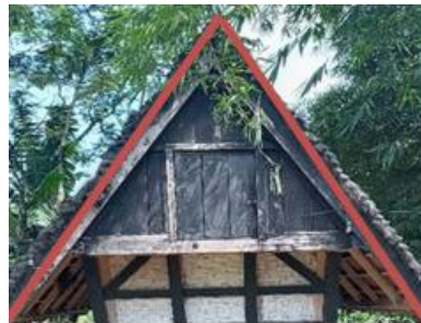
Figure 3. The part of roof
