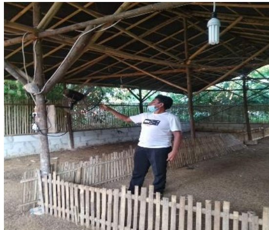
Figure 5. Cooling Fan Installation
