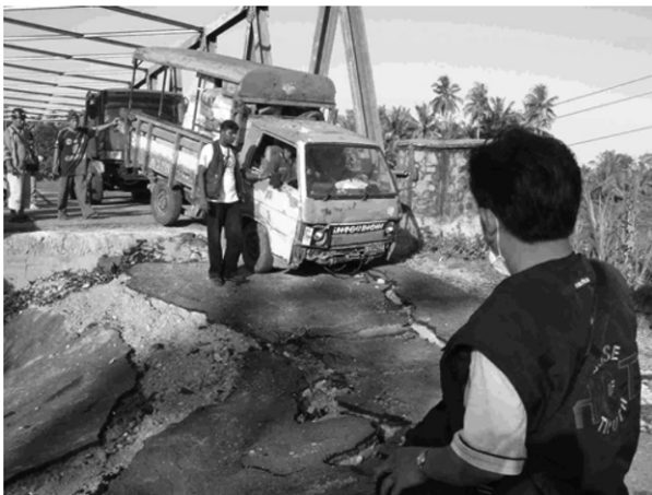
Figure 1. Maneuvering the truck through the damaged bridge.
