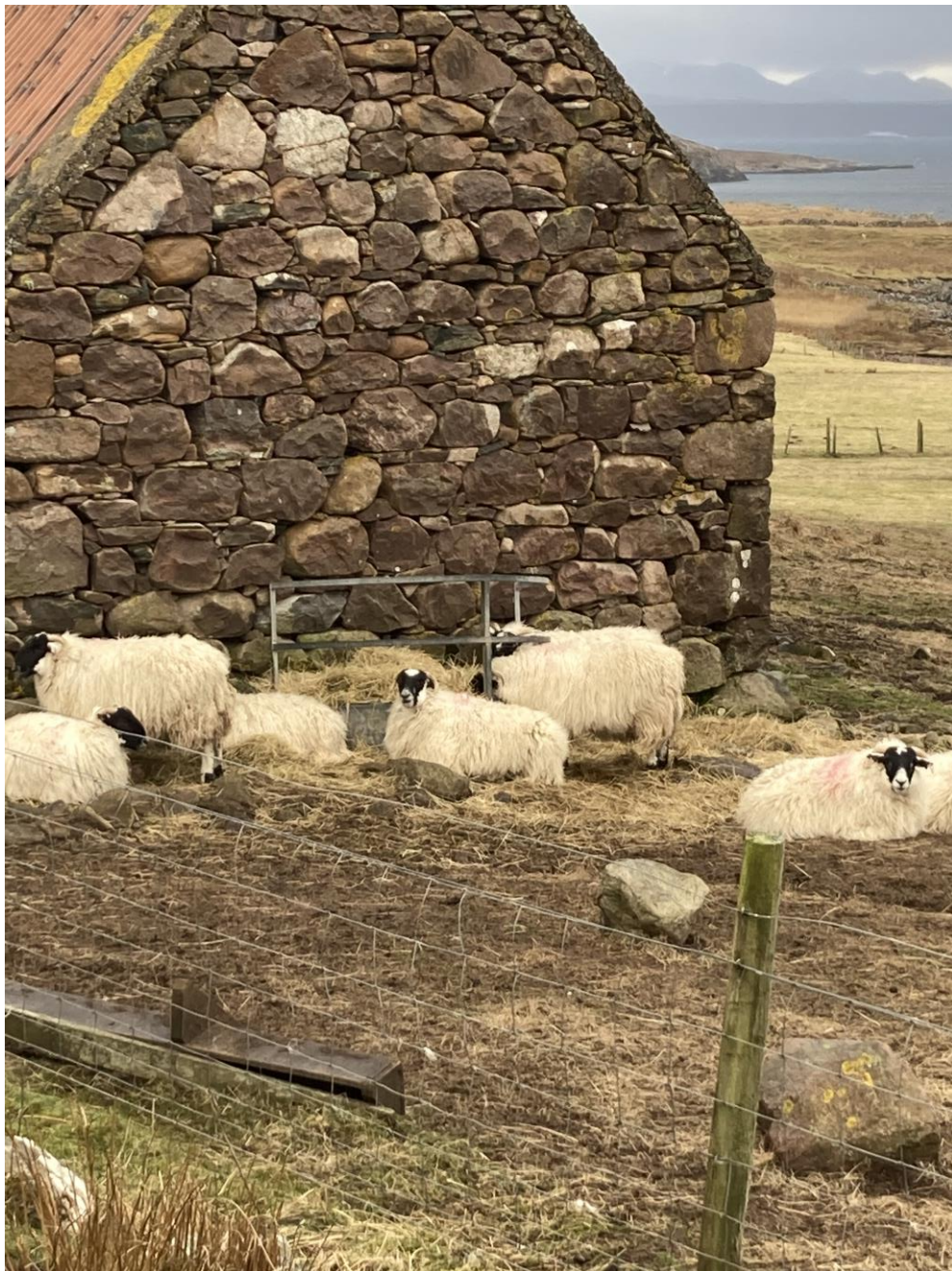
Figure 29: Shelter at a gable end
