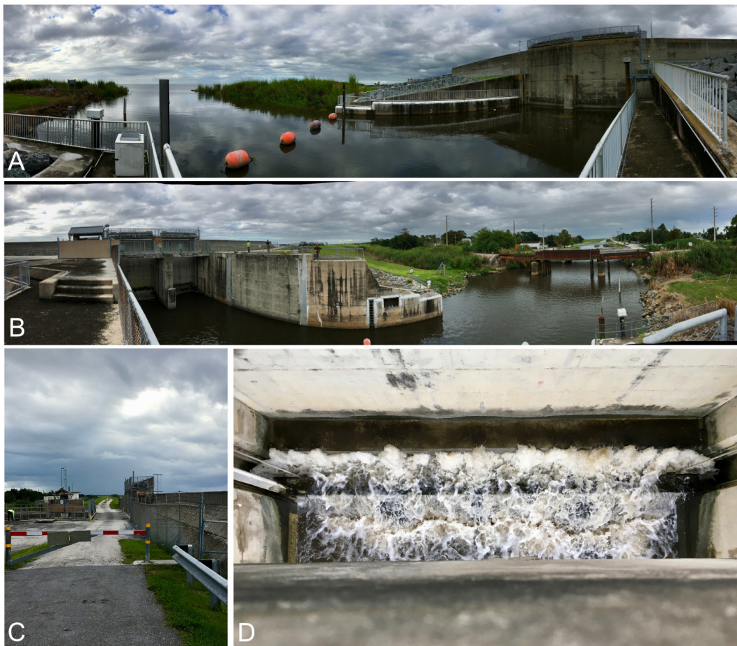
Fig. 7- One of several smaller water control structures (a dam) that discharge water from Lake Okeechobee to help maintain water levels. This structure is located on the West Palm Beach Canal at Canal Point on the Southeastern portion of the lake: A) a panorama of the lake side of the structure where water passively enters, B) a panorama of the canal side of the same structure where water discharges to the West Palm Beach Canal, C) the Lake Okeechobee Scenic Trail traversing the top of the dam, D) water discharging from the dam to the canal as viewed from the Lake Okeechobee Scenic Trail.
