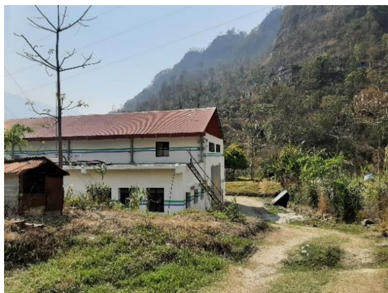
Figure 8. Small hydropower plant near Sunkoshi River, Nepal.
