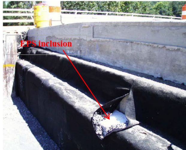
Figure 2.25 EPS inclusion in Jackson River Bridge, Virginia, US (Hoppe, 2005)
