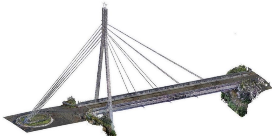
Figure 6. Generated point cloud of Werrington bridge.
