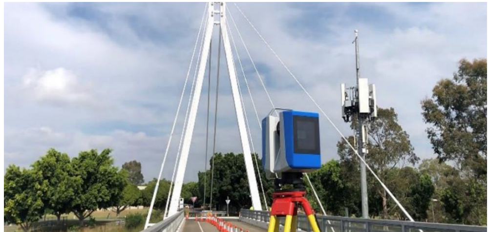
Figure 5. Laser scanning of Werrington bridge.
