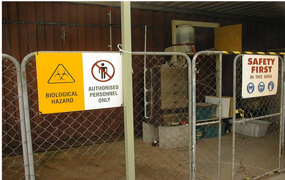
Figure 6.4 The test site was fenced and safety warnings installed.
