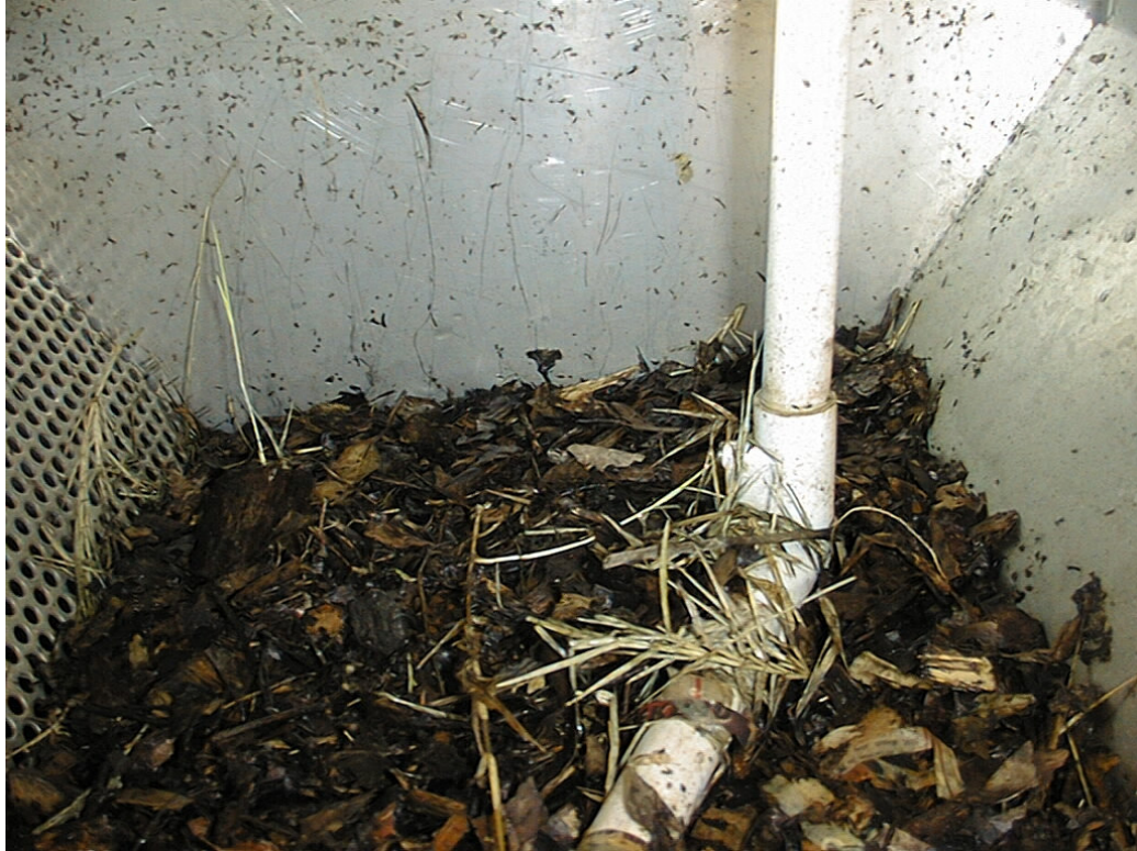
Fig II.8 Inside the upper compartment – V-hopper chamber
