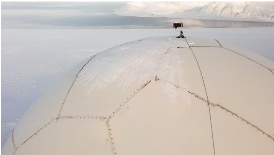
Figure 2.31: Example of snow on radome
