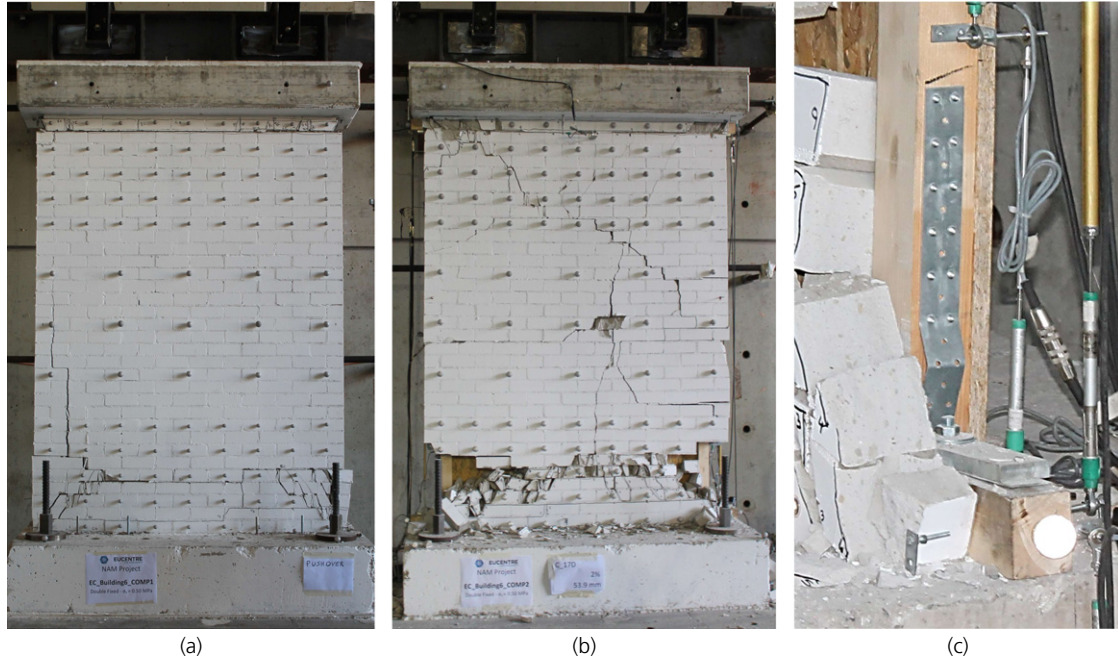
Figure 16. Ultimate conditions: (a) bare pier; (b) retrofitted pier; (c) buckled tie-down steel angle
