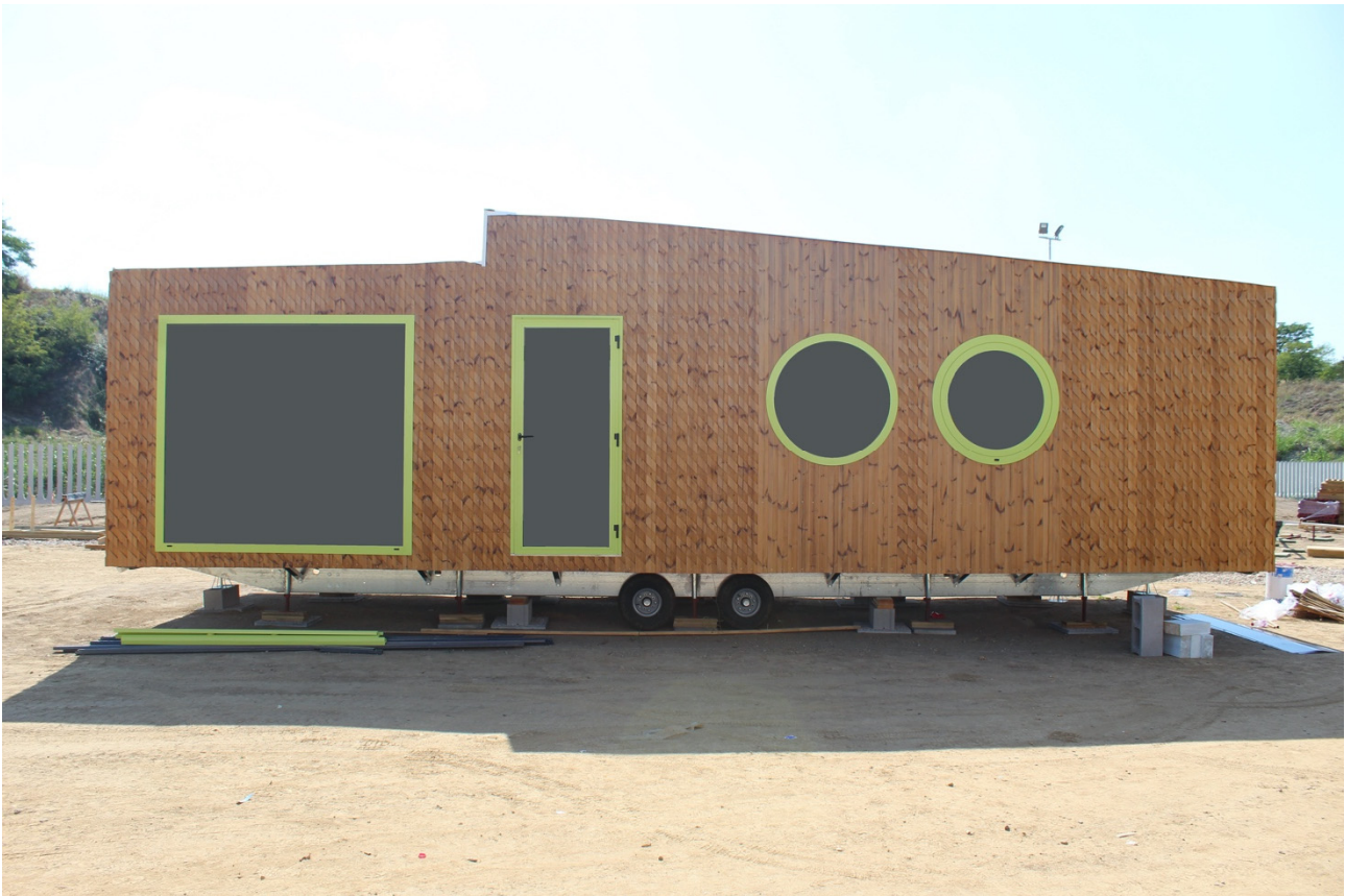
Figure 14. Picture of the prototype in phase of construction.
