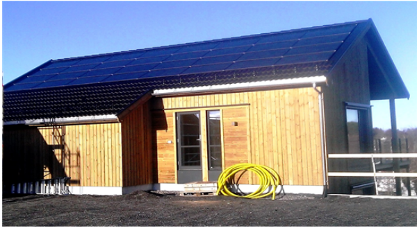
(b) Construction face picture of the specific studied house (C6) [14]
