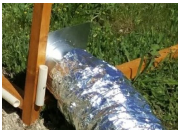
Figure 3. Picture of one of the circular openings of the greenhouse with a ventilation duct attached.
