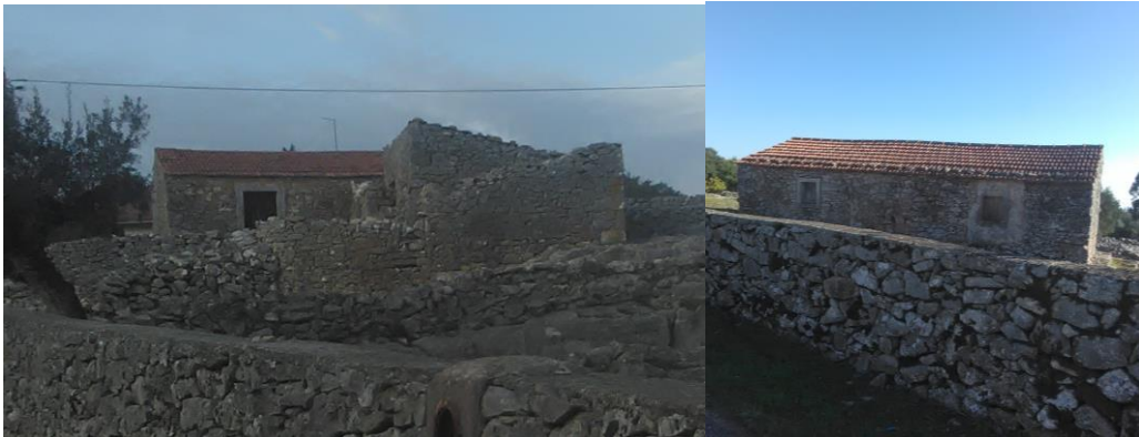
Pictures 75 and 76 - Pictures of building 16– Serra de Santo António
