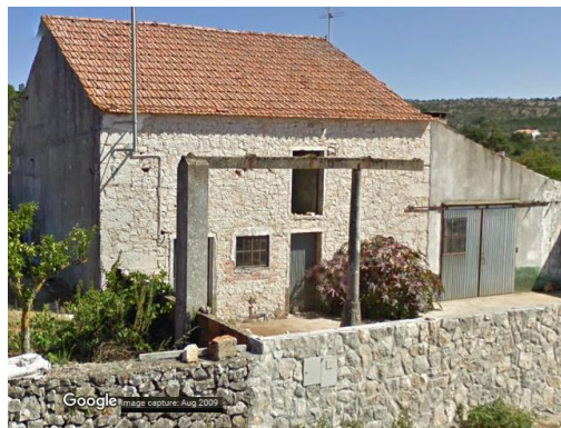
Picture 73 – Picture of building 15 in 2009 (google)
