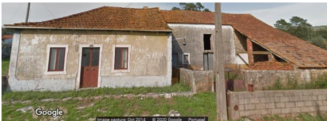
Picture 62 - Picture of building 11 in 2014 (google)
