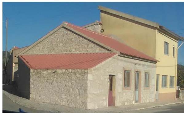
Picture 69 – Picture of building 14 – Serra de Santo António
