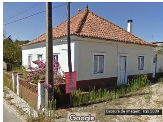
Picture 95 – Picture of building 22 in 2009 (Google)
