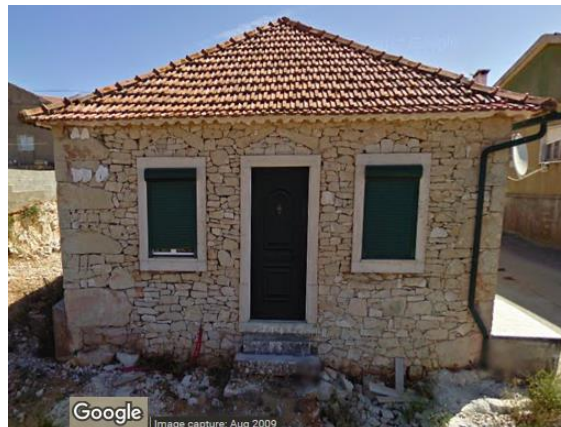
Picture 81– Picture of building 18 in 2009 (google)
