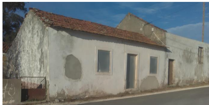
Picture 30 - Picture of building 2 – Serra de Santo António
