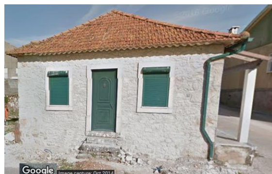
Picture 82 – Picture of building 18 in 2014 (google)
