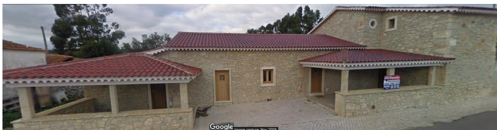
Picture 38 - Pictures of building 4 in 2009 (Google)
