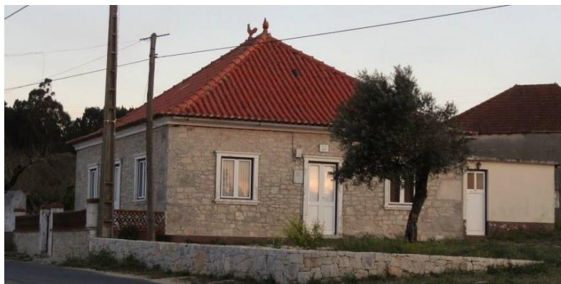
Picture 94 – Picture of building 22 – Serra de Santo António
