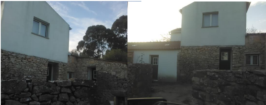
Picture 78;79 - Picture of building 17– Serra de Santo António
