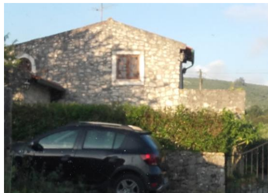
Picture 53 - Picture of building 9 – Serra de Santo António
