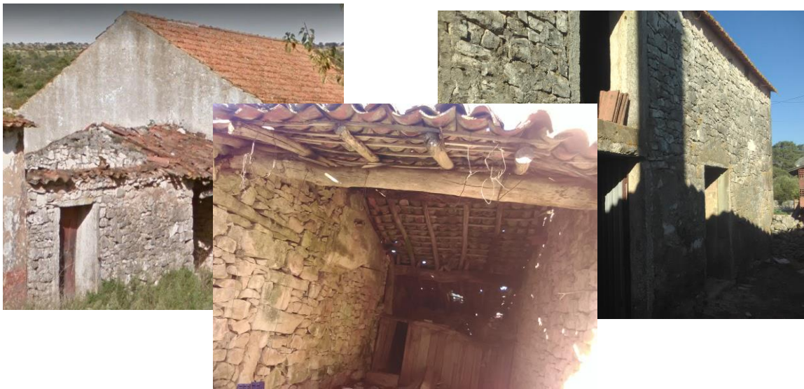
Picture 56-58 – Picture of building 10 – Serra de Santo António
