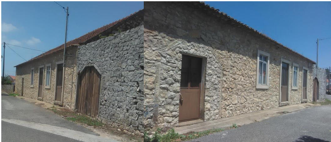
Pictures 91 and 92 – Pictures of building 21 – Serra de Santo António
