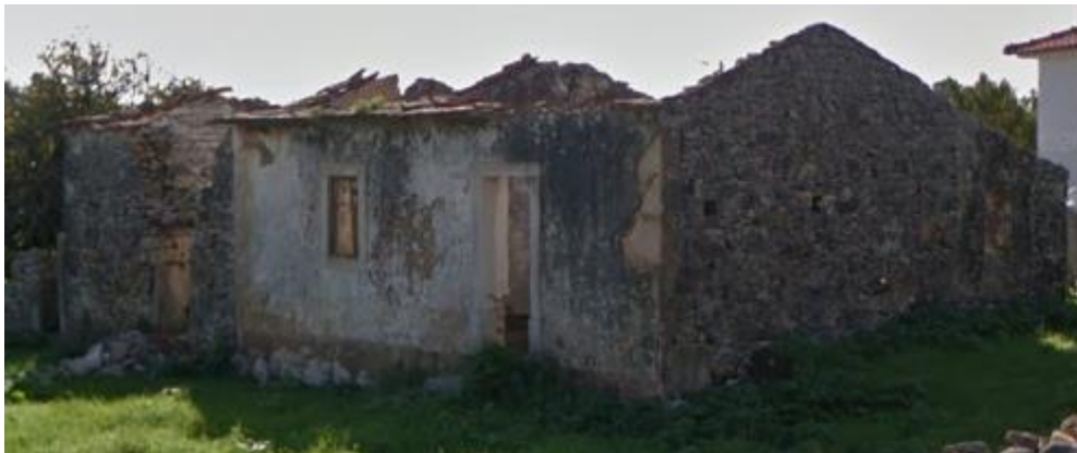
Picture 64 - Picture of building 12 – Serra de Santo António
