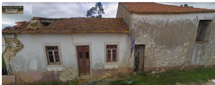
Picture 31 - Picture of building 2 in 2009 (Google)
