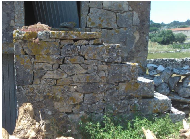
Picture 14 – Limestone stairs on the outside of building in Serra de Santo António
