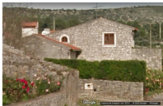
Picture 54- Picture of building 7 in 2014 (Google)
