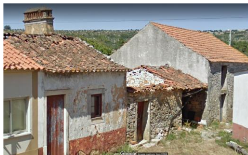
Picture 59 - Picture of building in 2009 (Google)
