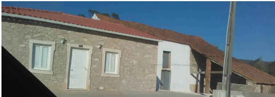
Picture 61 - Picture of building 11 – Serra de Santo António
