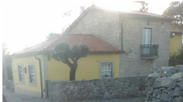
Picture 47 - Picture of building 7 – Serra de Santo António
