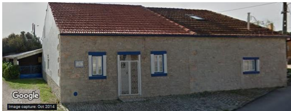
Picture 77 – Picture of building 13 in 2014 (Google)
