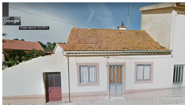
Picture 70 – Picture of building 14 in 2014 (Google)
