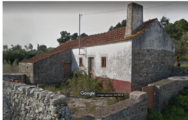
Picture 51 - Picture of building 8 in 2014 (Google)
