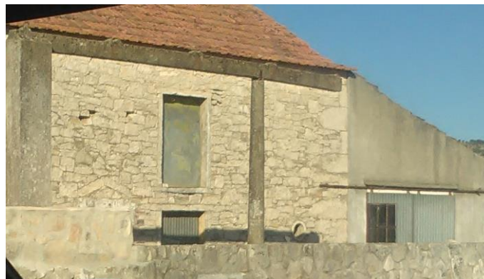
Picture 72 - Picture of building 15 – Serra de Santo António
