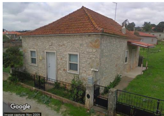
Picture 28 - Picture of building 1 in 2009 (Google)
