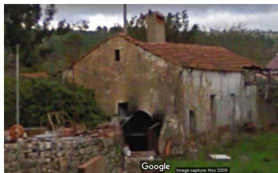
Picture 4 - Picture of building 3 in 2009 (Google)
