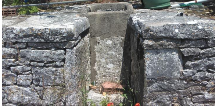
Pictures 8 - 9 – Pictures of limestone wells in Serra de Santo António.
