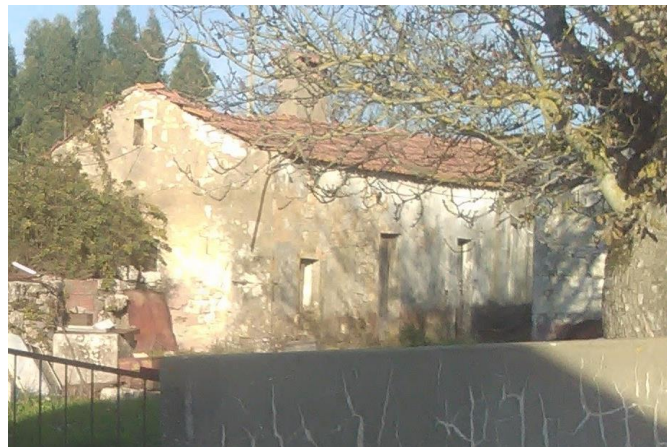
Picture 3 - Picture of building 3 – Serra de Santo António
