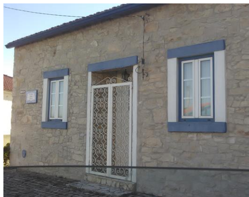
Picture 66 – Picture of building 13 – Serra de Santo António
