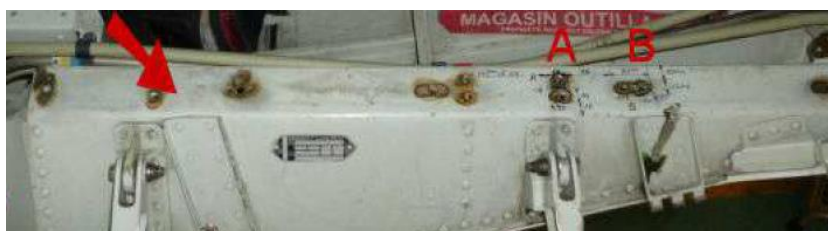
Figure 4.32: Superficial corrosion (light brown areas) found in mechanical servicing compartment floor beam. (Image obtained from NetJets Europe portfolio)
