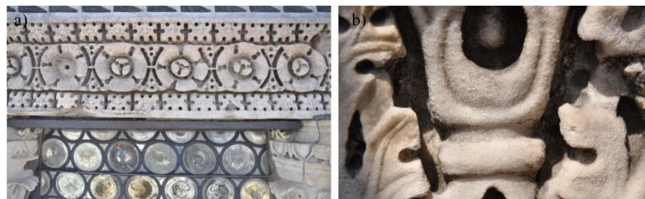
Figure 4. (a) An example of a widespread granular disintegration phenomenon (see detail in (b)).
