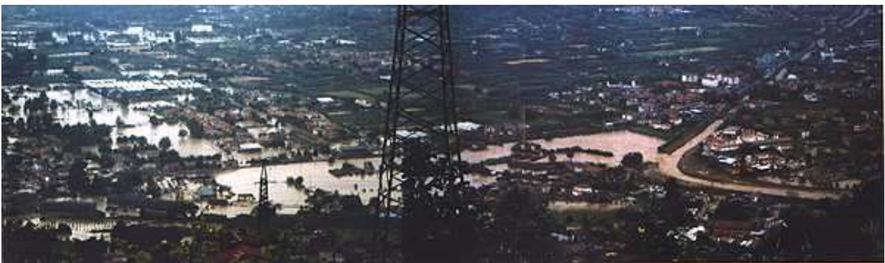
Figure 5.1 The flooding caused by the levee breach on 19 June 1996 formed along the Versilia River close to the town of Pietrasanta (source: http://www.neteservice.it/ilfiumeversilia/alluvione_Versilia96.htm ).
