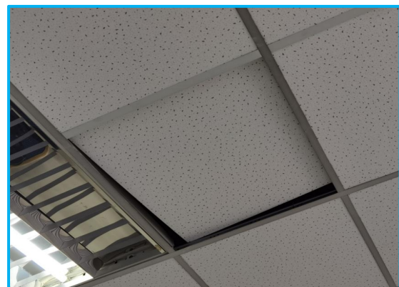
Figure 4.17: Four pieces of photos for architectural system minor defect
