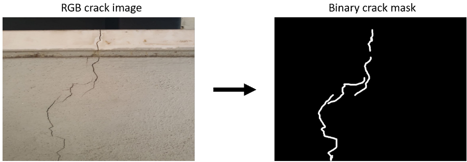
Figure 3.49: On the left the acquired RGB input image, on the right the binary model prediction
