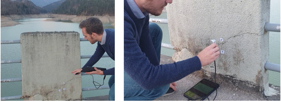
Figure 6.8: The bridge chosen for the inspections in conditions of natural light is located on the "Centro Cadore" Lake
