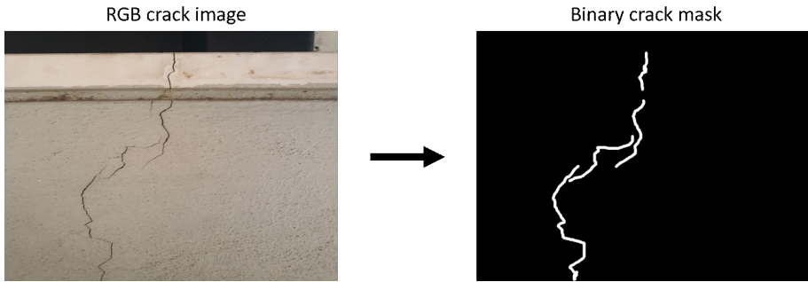
Figure 3.38: On the left the RGB crack image, on the right the binary crack mask manually selected by an operator.
