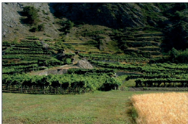
Figure 2. Example of terracing on alluvial fan of glacial origin made with the double aim to stabilize the slope and form surfaces where to cultivate grapes. Terracing faces southern exposure and spans from about 950 to about 1000 m above sea level. Morgex, Aosta, Italy.
